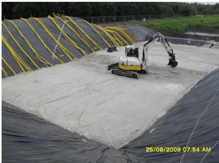
Figure E-3 the construction of the sand layer in de IJkdijk (de Bruijn, 2009)
