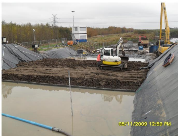
Figure E-4 the construction of the clay dike in de IJkdijk (de Bruijn, 2009)
